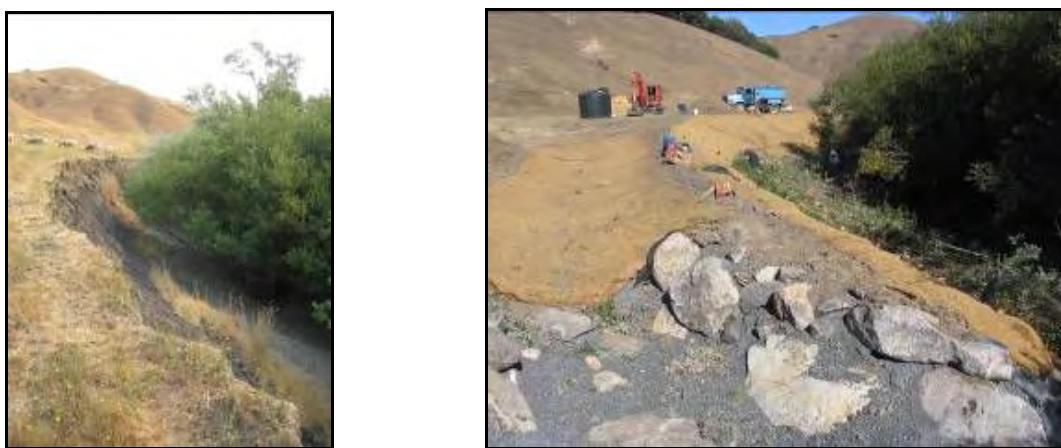
Figure 11: Photo-point sequence at a streambank stabilization project site pre-project (left) and during construction with installation of willow wattles following grading (right).
