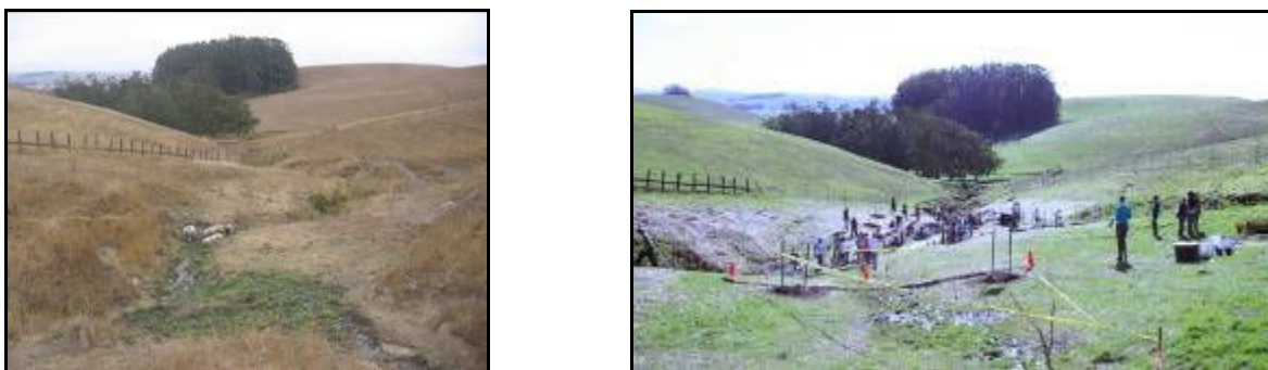
Figure 2: A gully site pre-project (left) and the STRAW revegetation day implementing critical area planting practice (right) following spring development and grade stabilization structures. Control fencing was constructed after the planting was completed.
