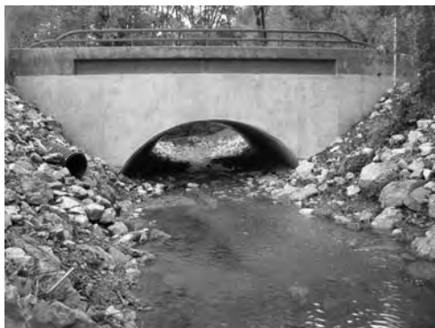
Arch culvert with natural stream bottom
