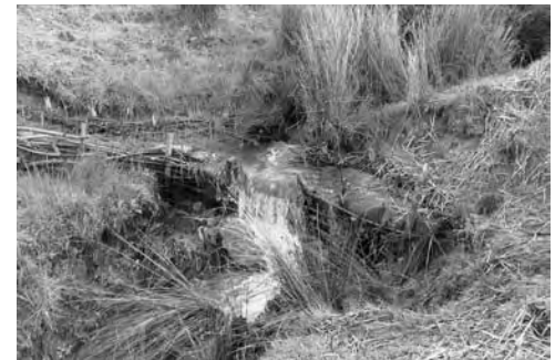
Willow wall headcut repair
