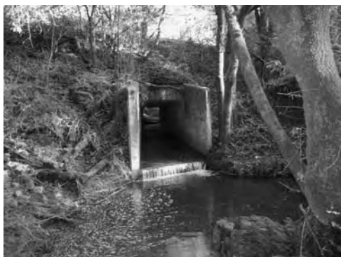
Traditional box culvert with concrete bottom
