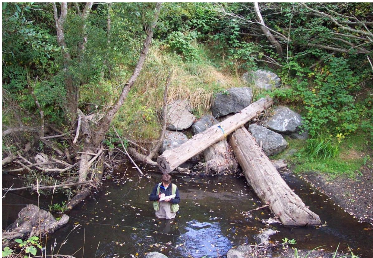
Figure 9. Numerous agencies, organizations, companies, and landowners are now adding large woody debris back into streams as shown here (two logs anchored with boulders). Photo by Karen Bromley.
