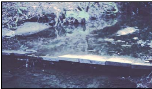
Figure 37: The first Stream Channel Improvement practice used a “Hewlett Ramp” design to confine high flows that scour deeper pools to improve habitat for steelhead and coho salmon. Designed by Prunuske Chatham, Inc and Trout Unlimited.
