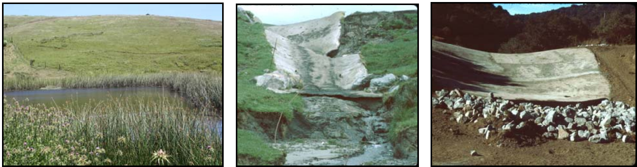
Figure 16: An example stockpond providing a critical source of clean water for ranch operations (left), failed spillway undermined by erosion caused by subsurface piping (middle) that was repaired by NRCS in 1985 and continues to function today (right). Photos by NRCS.
