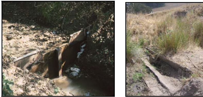
Figure 30: Examples of redwood board checkdams used as Grade Stabilization Structures with a recently constructed site in the 1980s (left), and a 30 year old site with deteriorated checkdam but vegetation such as Juncus has stabilized potential soil erosion (right). Designed by NRCS and Prunuske Chatham.
