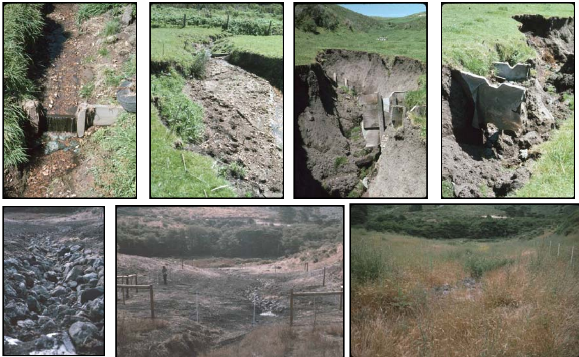
Figure 32: Photo monitoring of a grade stabilization project with functional redwood board checkdams before March 1986 storms (top left 2 photos), following March 1986 storms (top right 2 photos), the emergency repair installed a Lined Waterway with control fencing (bottom left 2 photos), and one year later in June 1987 (bottom right). Designed by NRCS.
