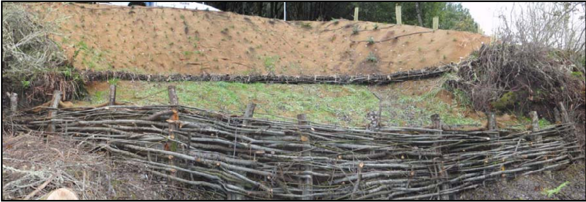
Figure 36: An example of the first willow walls constructed in 1990 in the Walker Creek Watershed (top), another later example constructed in 1994 (middle left), a recent design specification (middle right), and a recently constructed willow wall stabilizing the streambank toe below a threatened ranch road with willow fascine and revegetation using native grass seed, sedge/rush plugs, and shrubs in 2008 (bottom). Designs by Prunuske Chatham, Inc.
