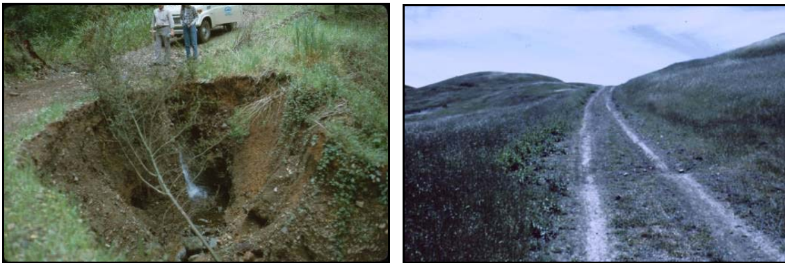
Figure 21: Examples of ranch road maintenance implemented in Lagunitas Creek Watershed following the 1982 flood in cooperation with Marin County Fire Department showing extensive erosion around a culvert outlet (left), and an upgraded road with out-sloped grade and water bar (right).
