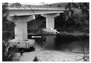
These bridge abutments were originally built at bed level
