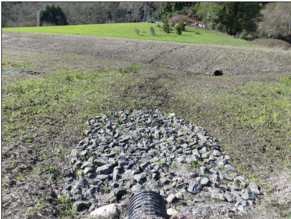
Photo Point 4: Looking west at rocked outlet.
