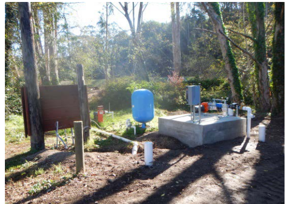
POD 2 for Pond 3B at SRF after Installation
