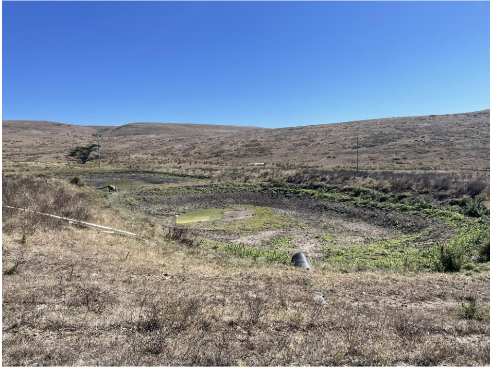
Below: Ponds 1 and 2, facing northeast.
