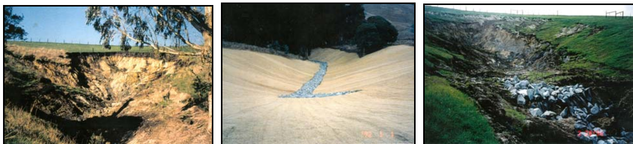
Figure 34: An eroding gully pre-project (left), after implementation of Lined Waterway and other practices in 1992 (middle), and four years later the site had unraveled (right).
