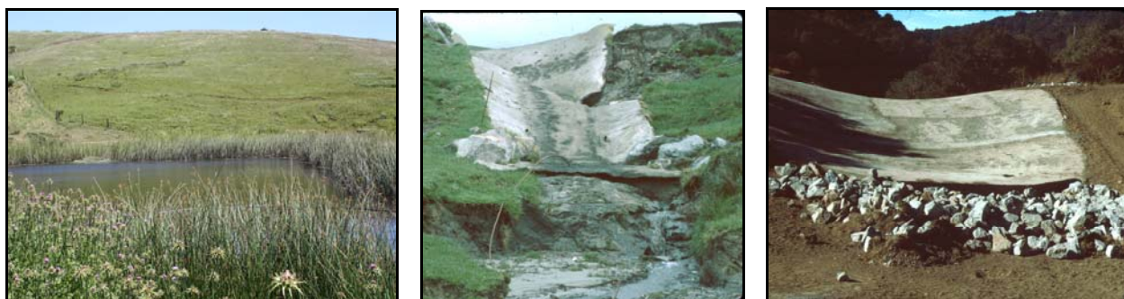
Figure 16: An example stockpond providing a critical source of clean water for ranch operations (left), failed spillway undermined by erosion caused by subsurface piping (middle) that was repaired by NRCS in 1985 and continues to function today (right). Photos by NRCS.
