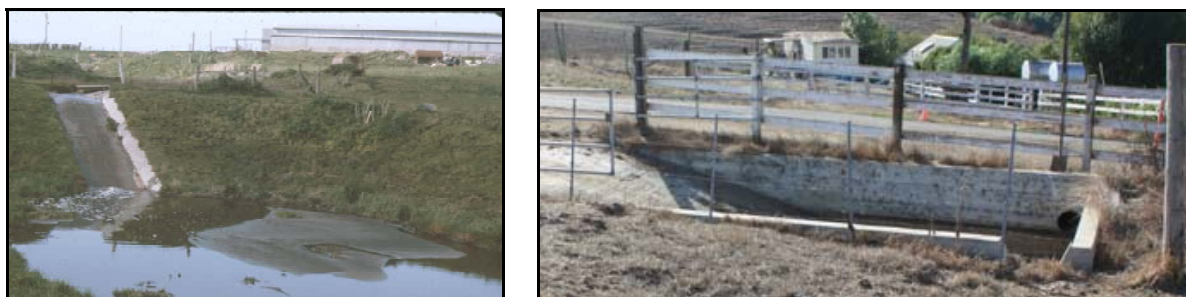
Figure 29: Examples of Sediment Basins depicting a large-scale design constructed in the 1980s (left), and a smaller version with a paved access ramp to facilitate maintenance built in 2005 (right).
