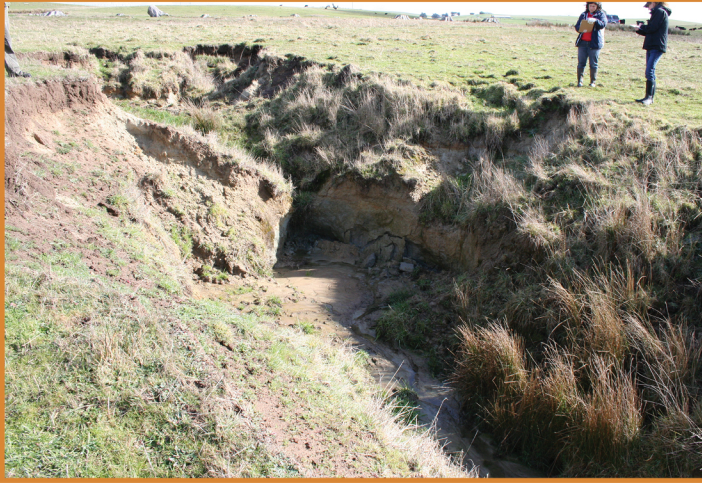
Marin Coast Ranch: A Series of Large Headcuts · PRE-PROJECT, 2012
