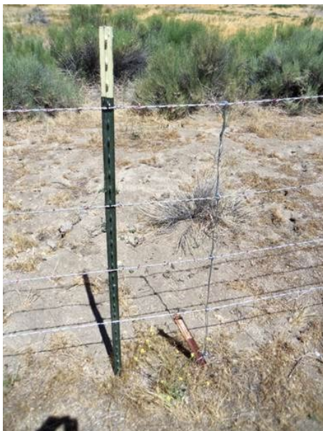
Earth-anchor used for change in topography and a break-away fence crossing a draw
