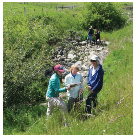
Marin RCD and partners fixed an eroding gully using bioengineered repairs. This reduced sediment and pathogen runoff and boosted wildlife habitat.
